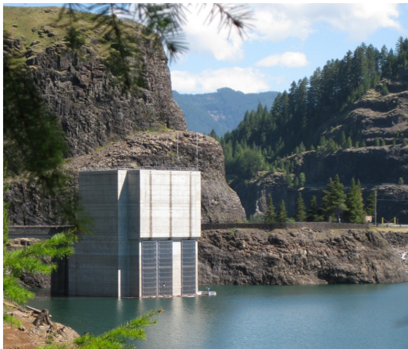
Figure 1. Photograph showing water temperature control (WTC) tower in the forebay of Cougar Reservoir, Oregon. Photograph by John Beeman, U.S. Geological Survey, 2010.
